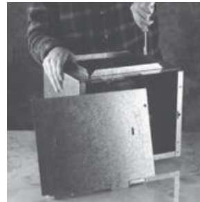
Step 2C. Install optional TDA panel and four screws.
